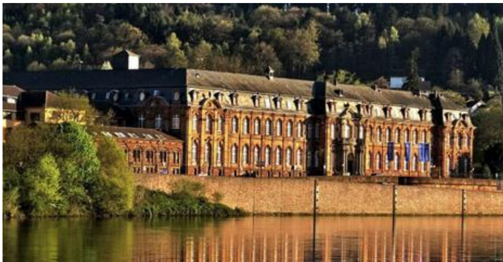
The Villeroy & Boch headquarters in Mettlach
